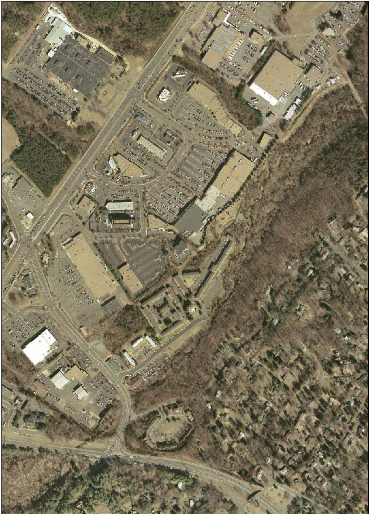
Figure AD 31: KMart Site Existing
