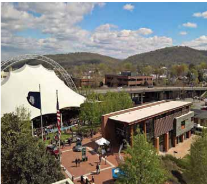
Figure 1. Downtown Charlottesville Transit Center
