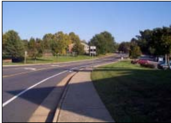
An example of an existing portion of sidewalk along Hillsdale Dr.
