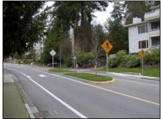
Median island with proper pedestrian markings.
