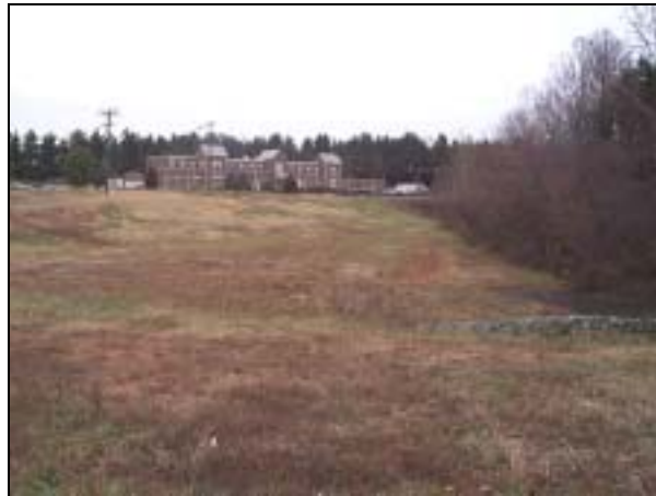
Stormwater detention area.
